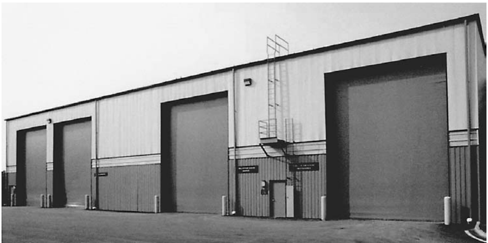
FIGURE 10.4 Large overhead doors are a staple of metal building systems. (Photo: Maguire Group Inc.)
